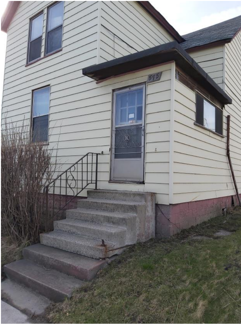
3. Front of building (North elevation).
