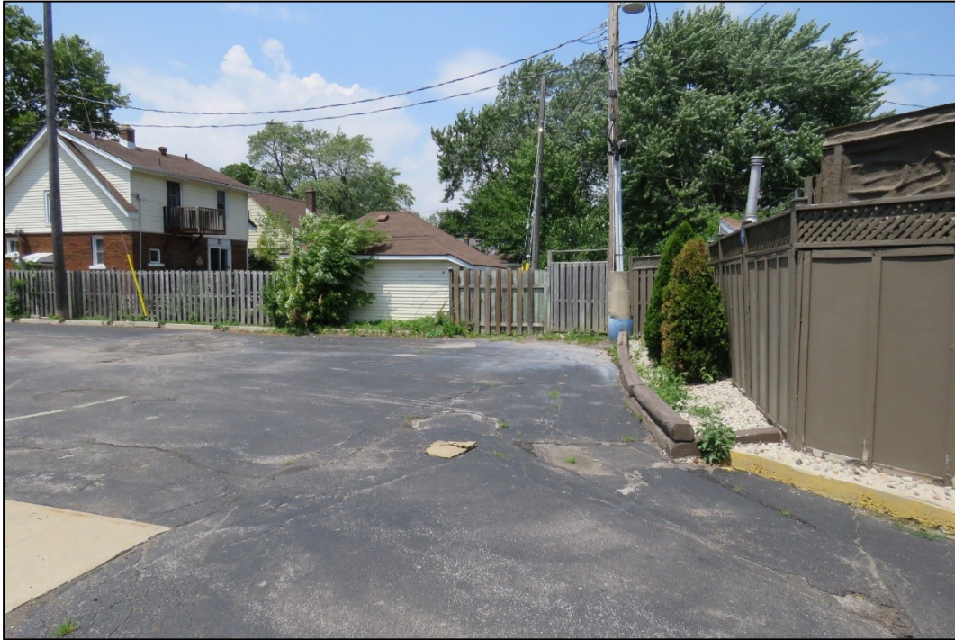
Figure 5 - Looking north towards encroaching landscaping feature in north/south alley
