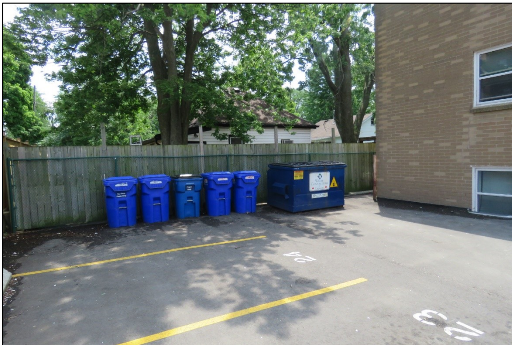
Figure 2 - Looking south towards alley from east parking area at 5335 Wyandotte Street East (alley located behind wood fence)
