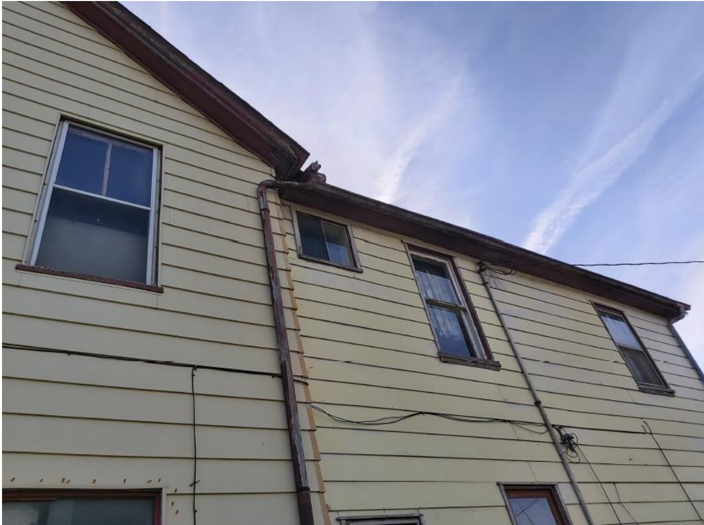
6. Side of building (West elevation).
