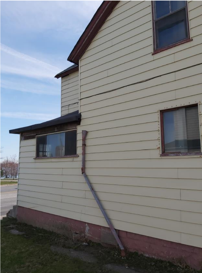
8. Side of building (West elevation).
