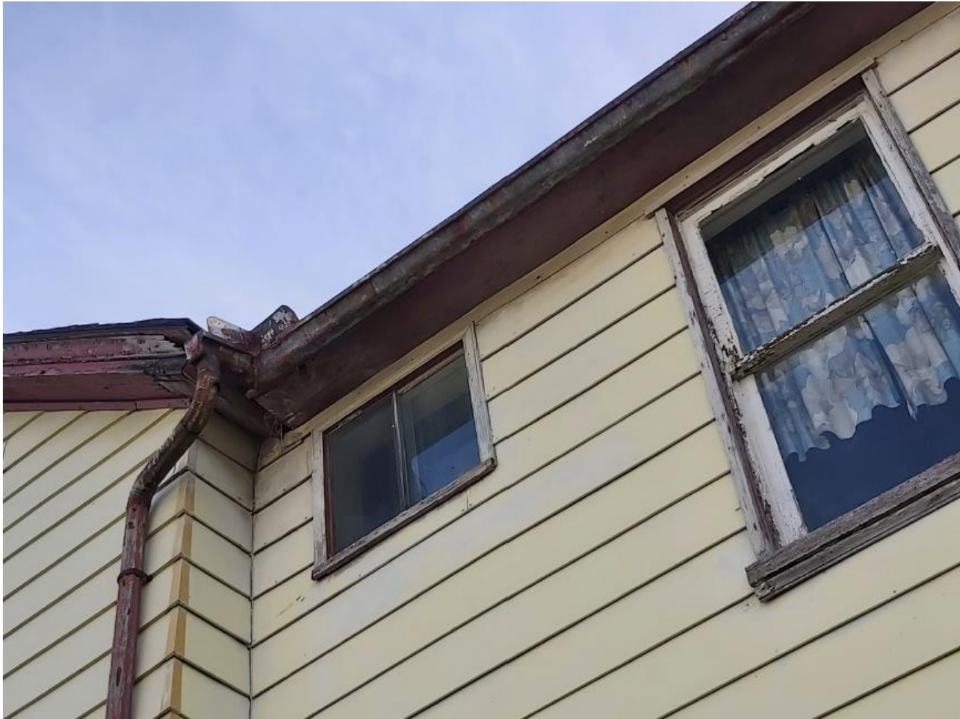
7. Roof line close up at side of building (West elevation).
