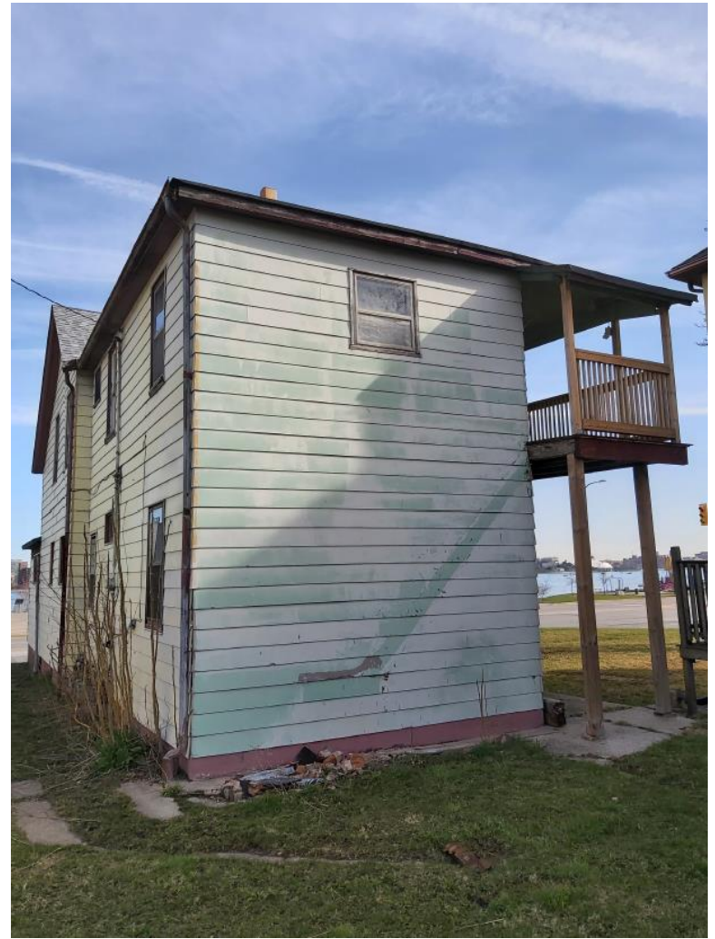
4. Rear of building (South elevation).
