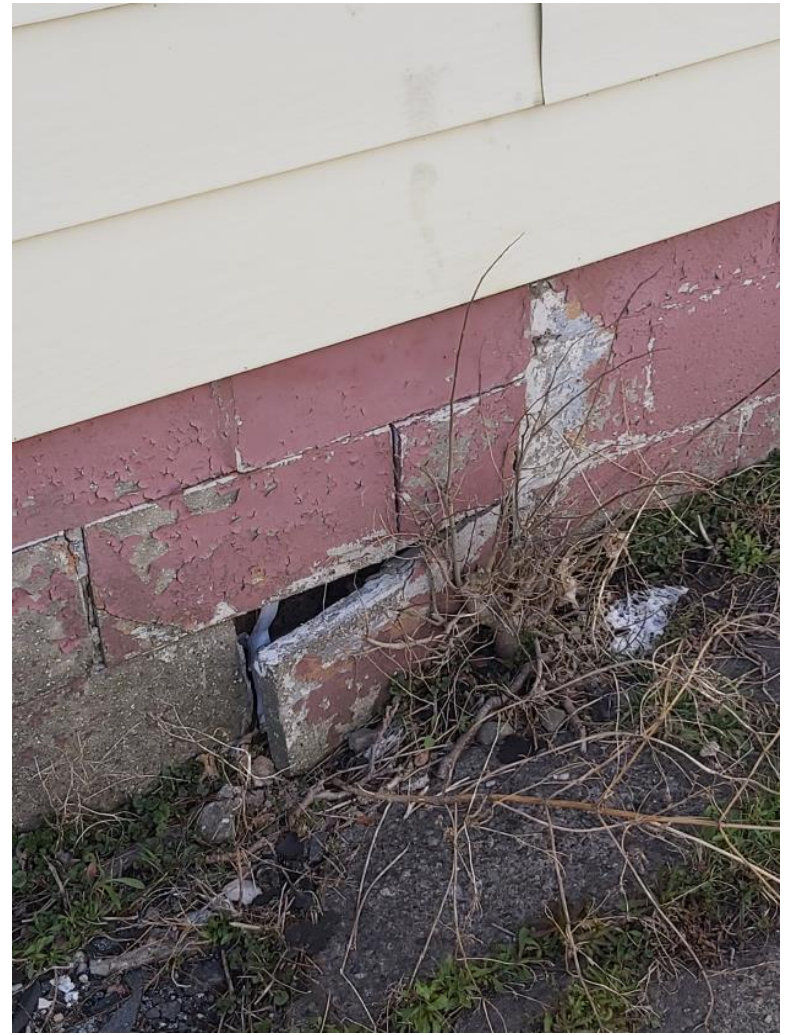
9. Foundation wall close up at side of building (West elevation).
